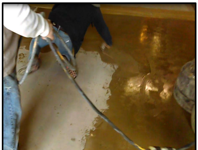
Installing grout; hand troweling is acceptable.
